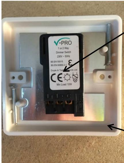
This is a module, in this form it can be removed from most dimmers
